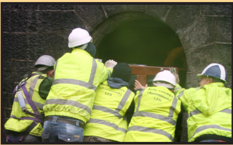
One final push sees the Pillar in!
