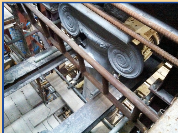
The final piece is put in place as the Ionic Capital stone is lowered and secured.
