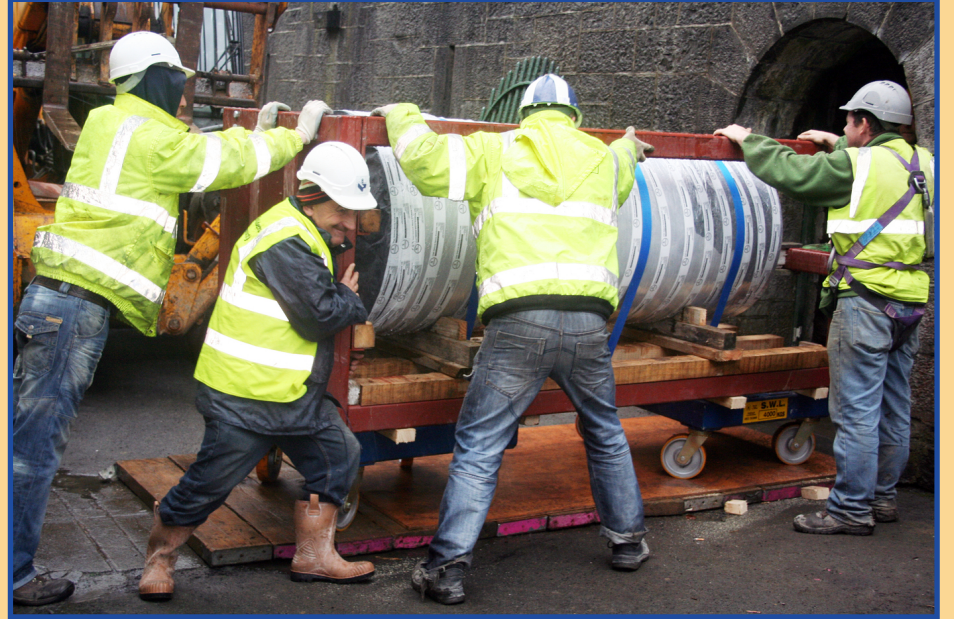
The replacement pillar is wheeled into the Crypt of the Cathedral manually.
