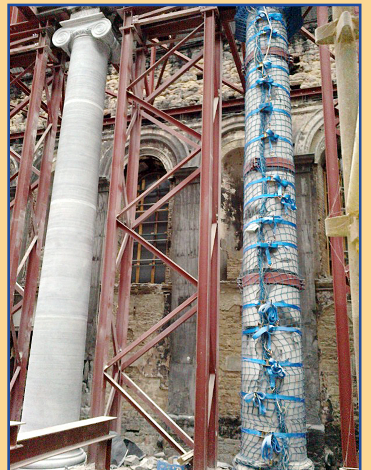
Picture shows the replica pillar in place alongside fire damaged pillar.
